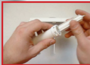
INSTALL STEP 4 Insert safety valve correct side
