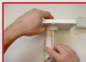
INSTALL STEP 5 Insert the tee-piece till the end
